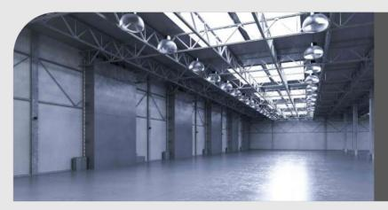
**Steel joist girders** are installed in roofs and floors to assist with the weight distribution of the structure. They are bolted to the columns and are installed fast and easily, which will also save you time and money on labor costs.
