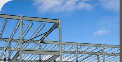
Load zone joists are installed in certain areas of the building in which more strength is required to provide support to the structure.
